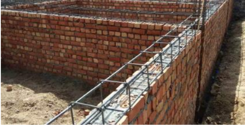
Figure 169: Pouring of concrete into the formwork
