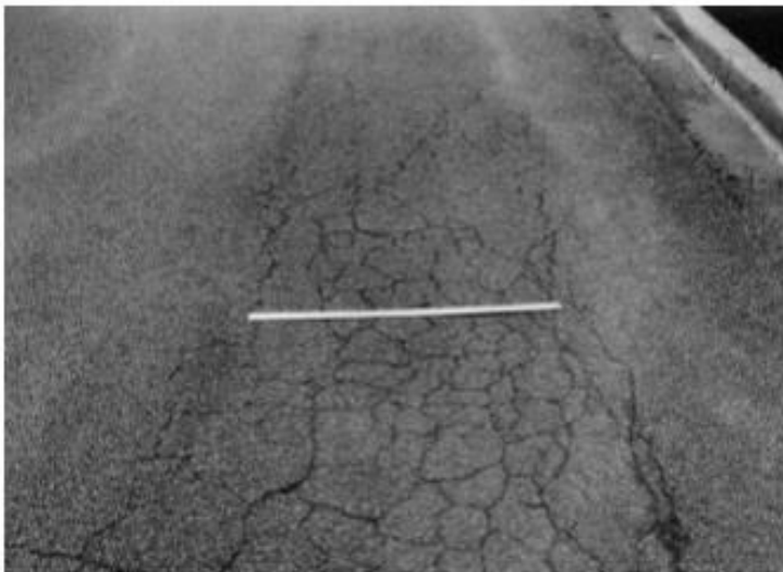
Figure 138: Alligator cracking
