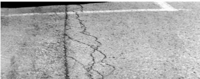
Figure 142: Edge cracking
