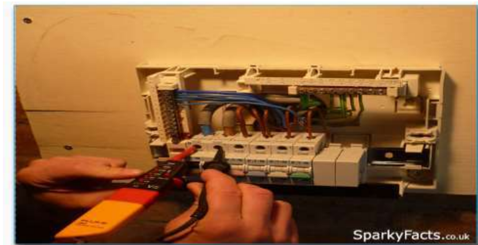
Figure 312 Test between Line and Neutral terminals
