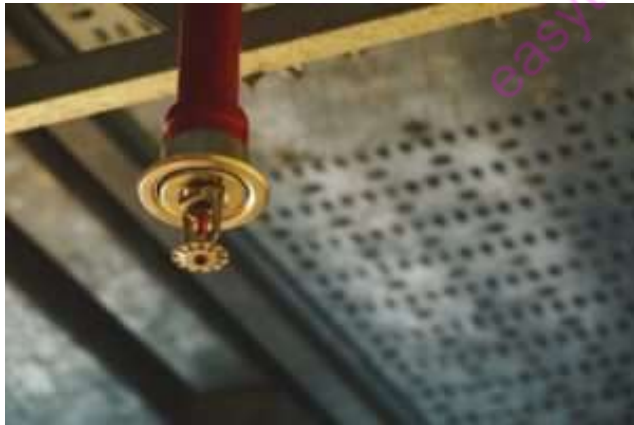
Figure 191 - sprinkler head
