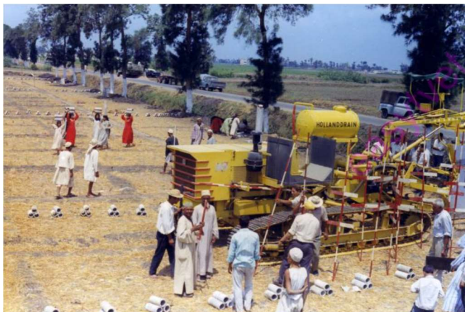
Site clean-up in action
