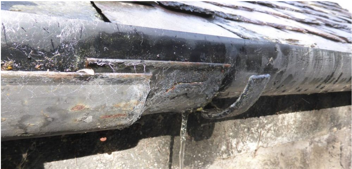
Figure 160: gutter brackets
