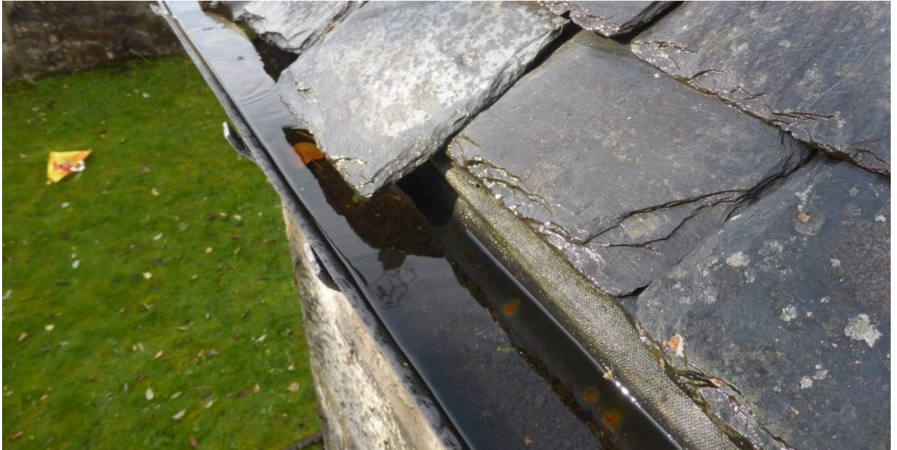
Figure 159: Blocked downpipes
