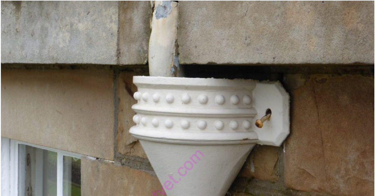
Figure 161:Downpipe brackets
