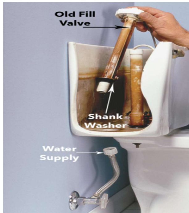
replacing old toilet fill valve
