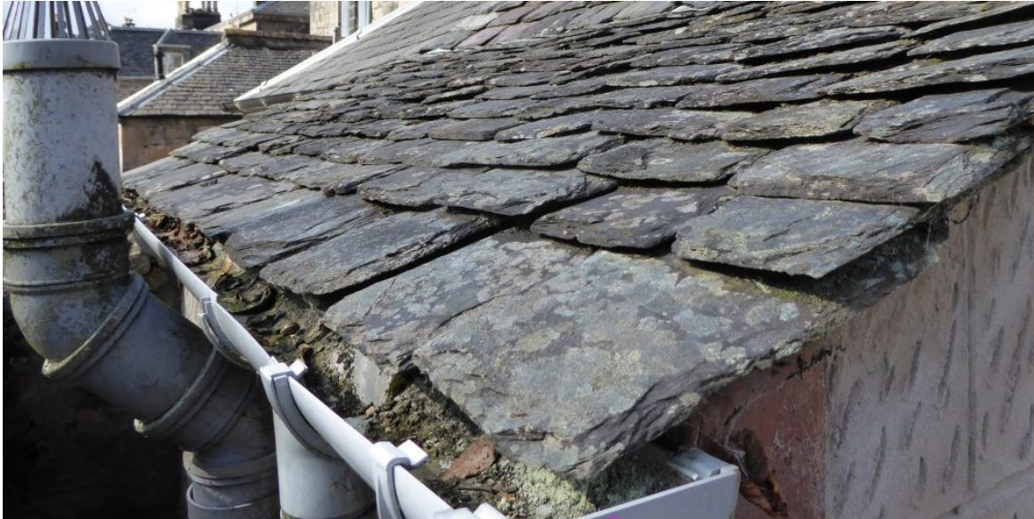
Figure 158: blocked gutters
