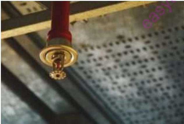
Figure 191 - sprinkler head
