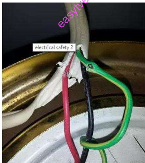
Figure 3: damaged insulation
